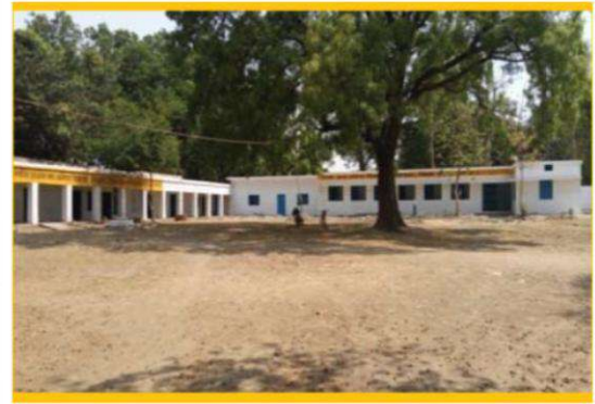
Renovation of Hr. Sec. School at Sijhata
